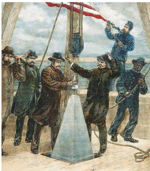
Setting the aluminum cap on the Washington Monument in 1884. At that time, aluminum was regarded as a precious metal.
