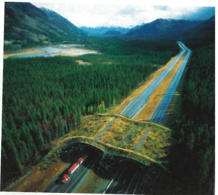
FIGURE 16.13 By providing a safe way to cross barriers such as roads and highways, land bridges such as this one in Canada allow animals to move safely from one part of their habitat to the next.
